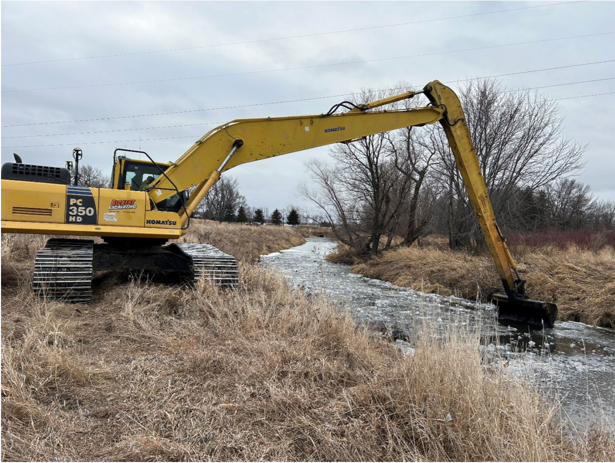
Figure 1. Cleanout at Lake Allie Desilting Basin (November 2024)
